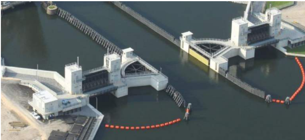
Figure 4.1: Example of sector gates and sluice gates (New Orleans)
