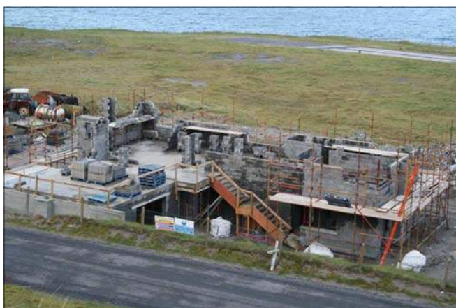
New health centre being built on Inis Oírr
