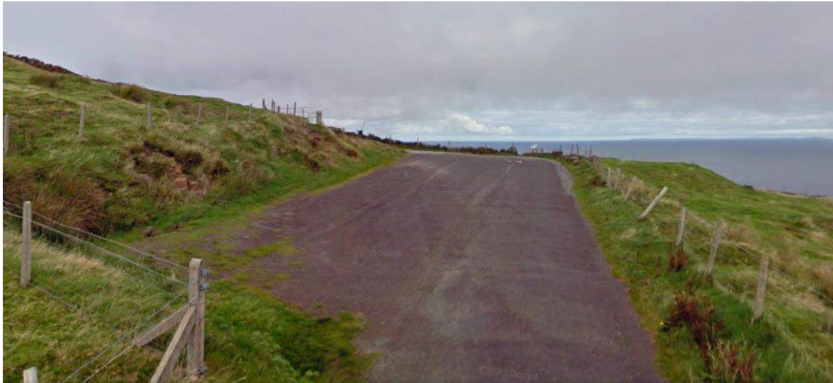
Fig 4.6 Limited car parking space at Brandon Point and no 'lined' car parking spaces. No turning point for coaches.
