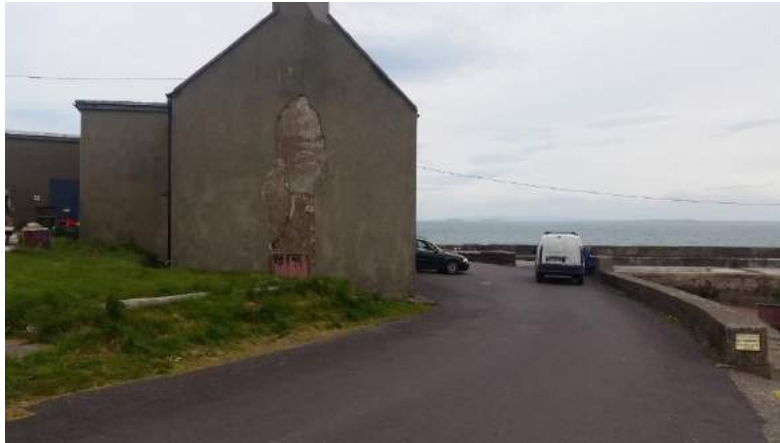
Fig 4.3 No car space marked out at Brandon Pier leading to vehicles being parked at all angles.
