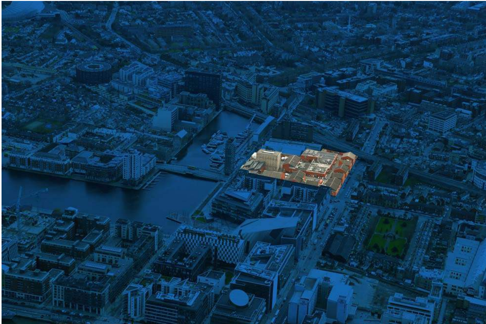
Location for Trinity Technology and Enterprise Campus and the Innovation District Dublin – Silicon Docks
