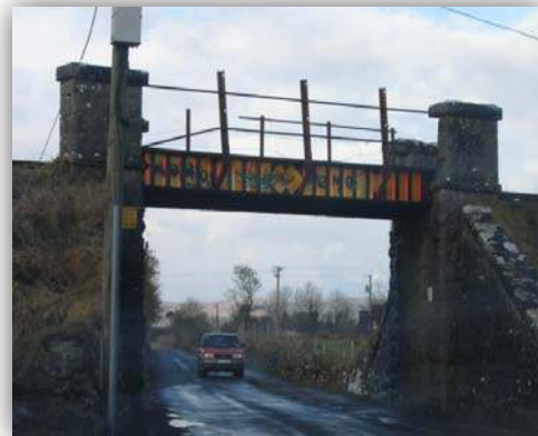
Photo 10 Railway Underbridge at Tubbercurry
