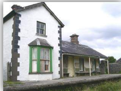
Photo 3 Leyney Station (Source: NIAH)
