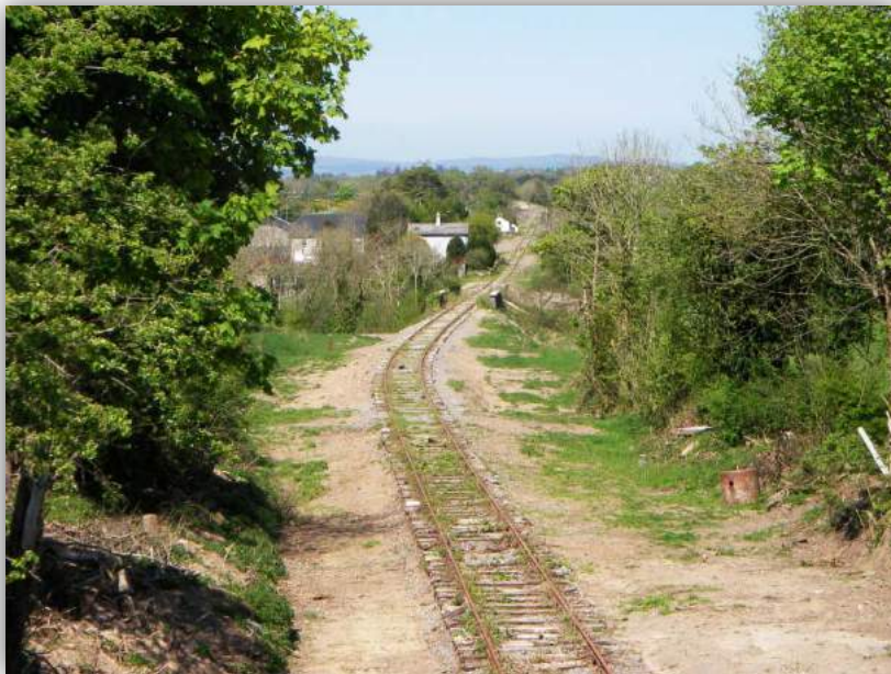
Photo 16 View North from Curry (copyright: West-on-Track)
