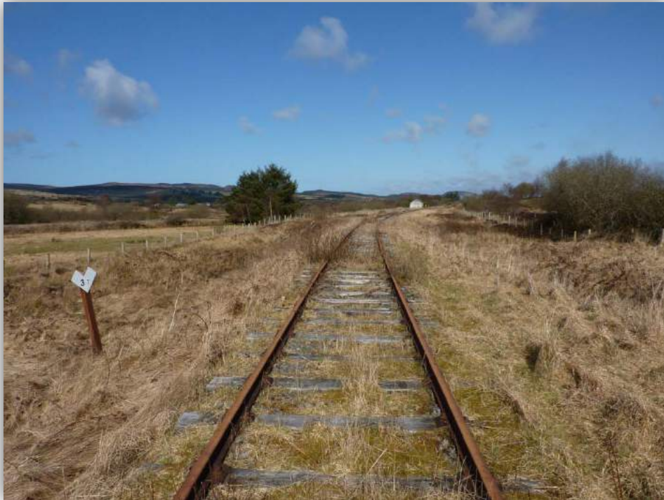
Photo 13 Looking Northeast towards Carrowloughan (copyright West=on=Track)
