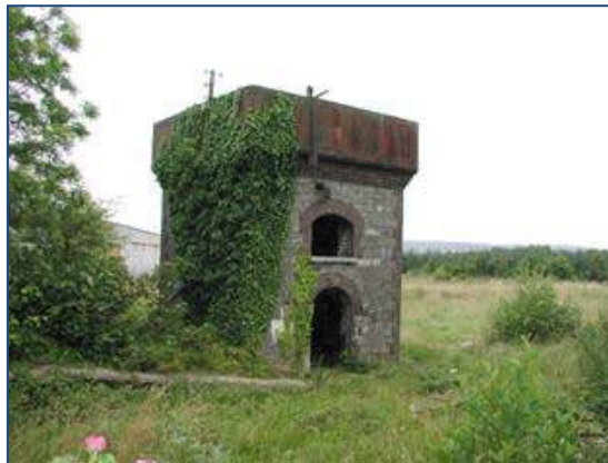
Water Tower at Tubbercurry (source: NIAH)
