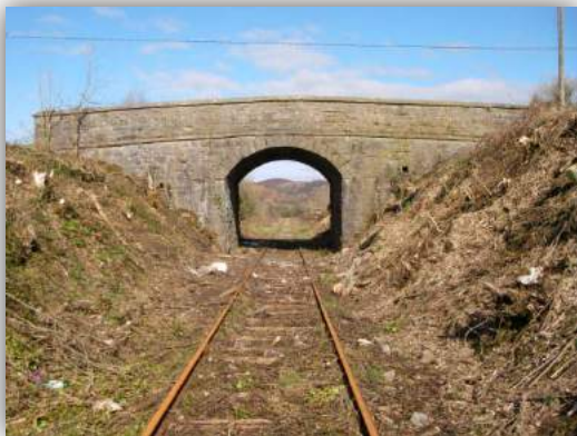
Photo 9 Railway Overbridge (copyright West-on-Track)
