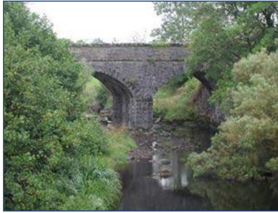
Railway Bridge at Curry, c.1890 (source: NIAH)
