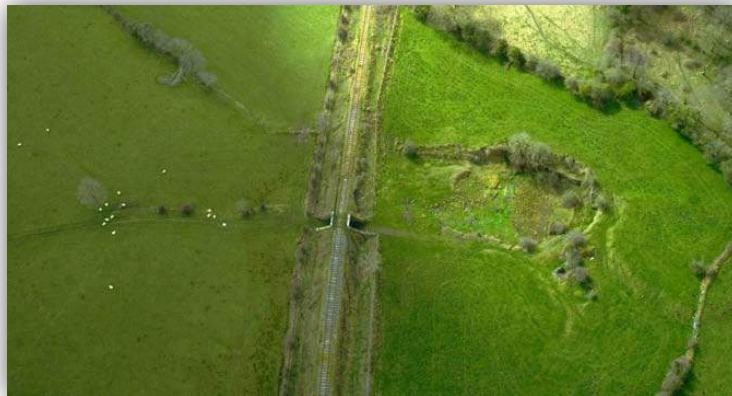
Photo 7 Aerial View of Carrowleam Underbridge (source: Irish Rail)
